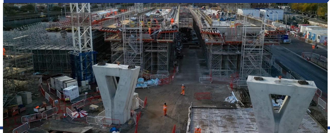
Curzon Street, Birmingham
