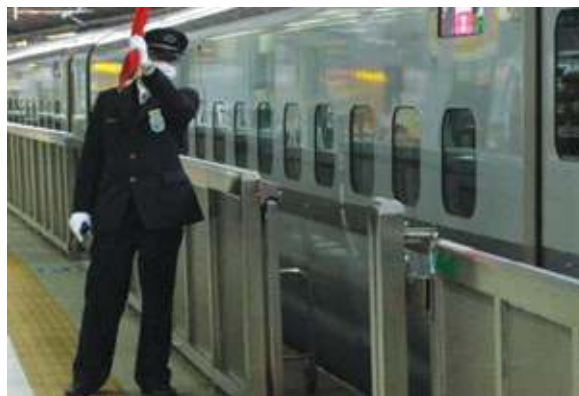
FIGURE 10, Platform gates
