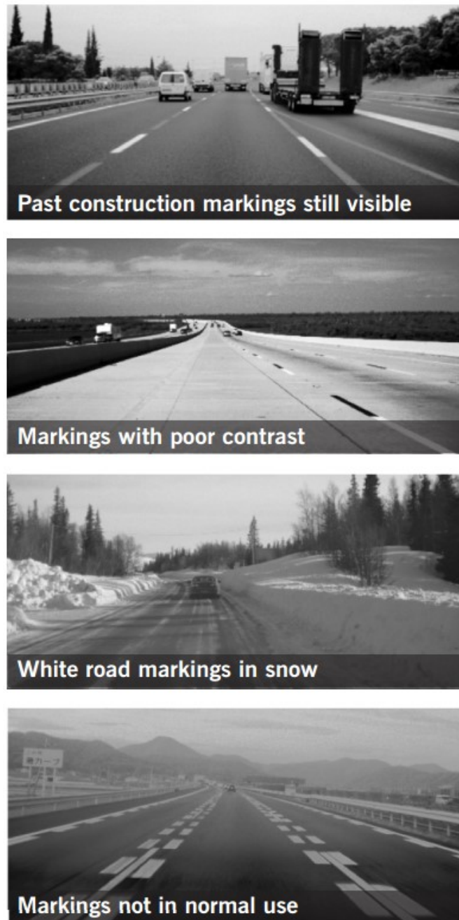
Figure 14: Failure Modes and Limitations, Extract from 'Roads that Cars can Read – A Consultation Paper', ERAP
