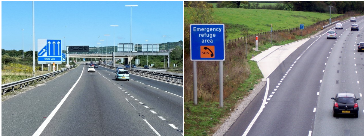
Figure 18: Example of continuous hard shoulder (left) and Emergency Refuge Area (right)
