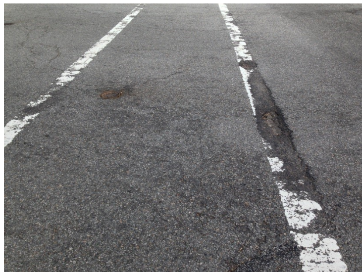
Figure 16: Example of poorly maintained road markings that may be difficult for CAVs to interpret [Source: https://upload.wikimedia.org/wikipedia/commons/f/f1/Road_surface_deterioration_by_pavement_markings.jpg ]
