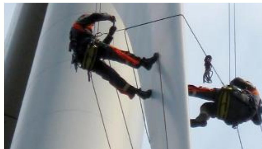
Rope access inspections are typical
