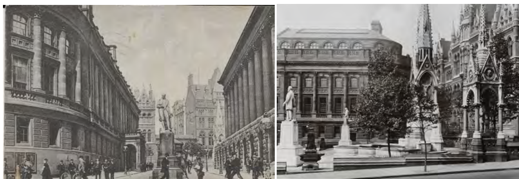
Left: Midland Institute & Birmingham Library (demolished 1974) looking towards Chamberlain Square with the Town Hall on the right.
